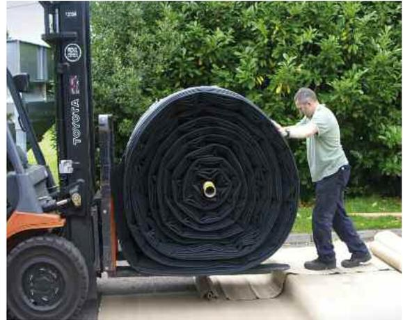
A 1.00mm Greenseal Geomembrane 26m x 53m being prepared for use as a dirty water lagoon at a dairy farm in Taunton.
