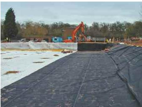
Greenseal Geomembrane being installed for a reed bed (Rockwood).
